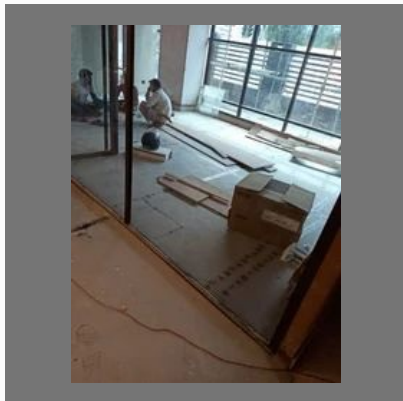
Floor Guard Sheet- TEMPRORY FLOOR COVERING
